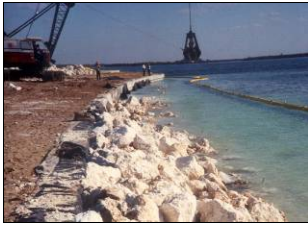
Erosion Control/ Bulkheads
