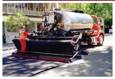
Asphalt overlay fabrics can extend the life of all existing paved areas. These specially manufactured nonwoven geotextiles are first saturated with heated liquid asphalt during installation, and creates a moisture barrier between old and new pavement. In addition, they absorb stresses to retard reflective cracking, thereby improving and extending the overall performance of the new overlay.
