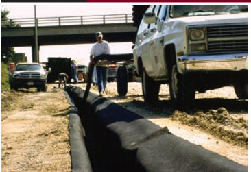
This is one of the most common applications of geotextiles in the construction of roadways, landfills, athletic fields etc, allowing for rapid removal of water or other fluids while providing excellent soil retention, assuring long-term free flowing drainage.
